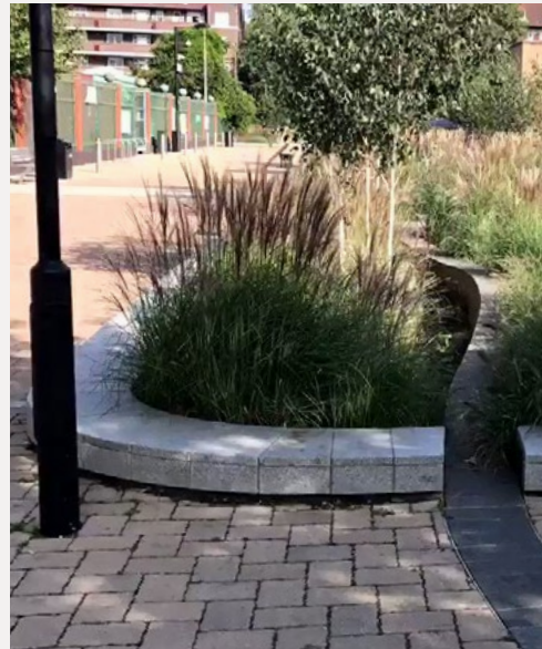
Planting schemes double up as sustainable urban drainage that can harvest and retain rainwater from peak rainfall for use at drier times of the year. Credit: Robert Baray Associates
