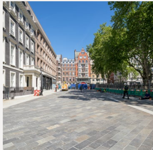
Extended and decluttered forecourt at the Bond Street station entrance with special paving creates a decluttered environment. Credit: Edward Bishop
