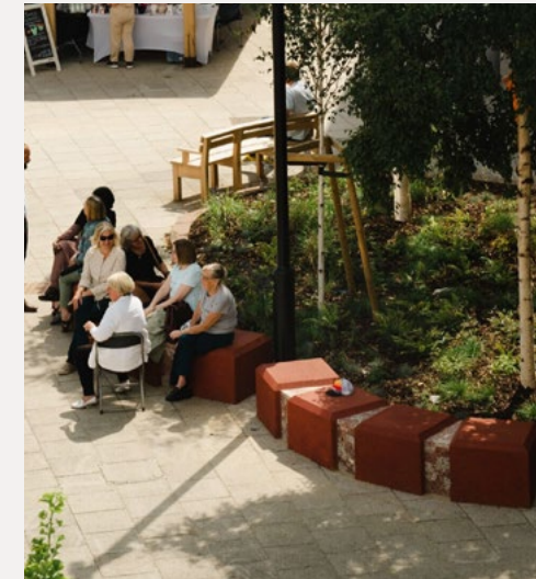
Existing concrete bollards in Bermondsey Blue Market were stained in red and repurposed to form continuous seating. Credit: Hannah Thual
