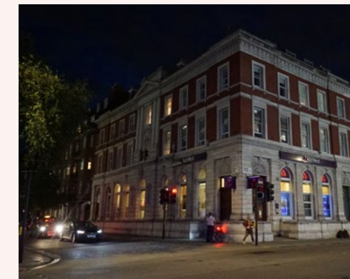
The corners on Baker Street are not active at night, lined with banks, estate agents, and other retail shopfronts
