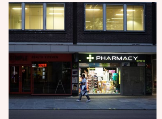
Some architectural and retail lighting is very bright, making other parts of the street seem dark in contrast
